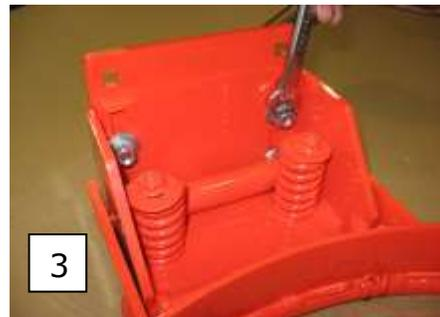
5. Insert bottom two carriage head bolts into place and finger tighten using flatwashers, lockwashers and hex nuts. (Add flatwashers, lockwashers and hex nuts if threaded studs are located at lower attachment points)
