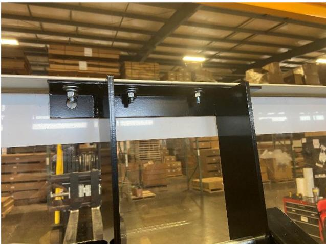
14. Loosely attach backboard to H-Frame at the four points along the bottom of the backboard frame as well. Use the 5/16" hardware provided in the bolt kit. Remember, IF YOU HAVE AN ACRYLIC BACKBOARD, make sure to get the gasket sandwiched between the backboard and the face of the H-Frame. (We recommend tape to hold it in place during assembly) Also, be sure the holes in the backboard and the holes in the H-Frame are aligned so the rim bolts will
